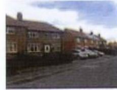
Station Road : existing houses to the North of the site
